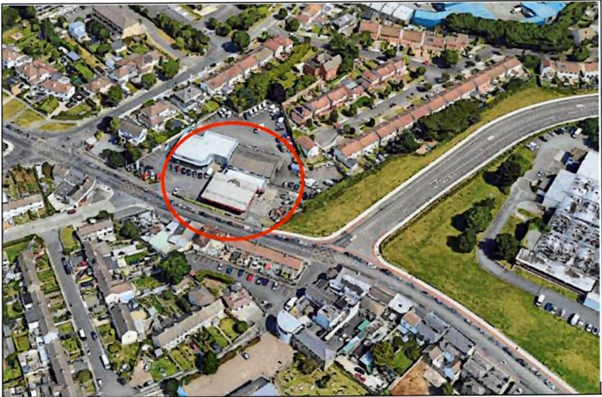
Figure 2 – View of Service Station in relation to surrounding context (Source: Google Maps, 2023)
